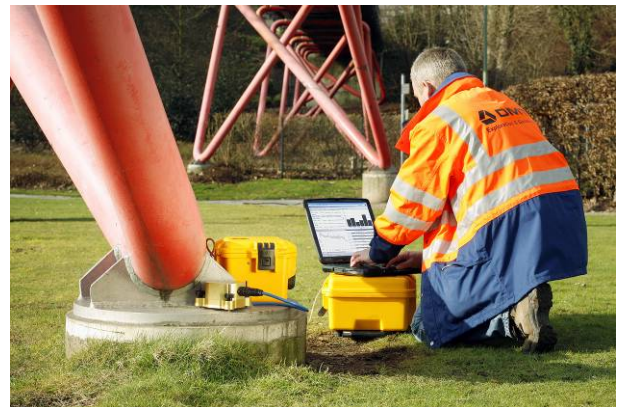
Monitoring of footings
